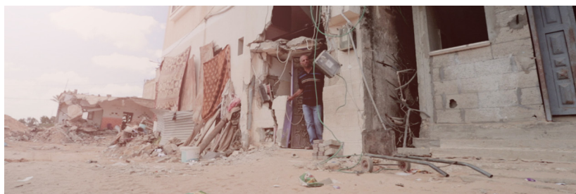
Mu'en Fayeز Qdeih (39), in front of his house that was damaged by Israeli strikes
